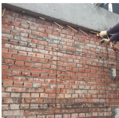
(c)彎折剪力連結筋
