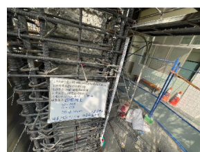
鋼筋綁紮及植筋
