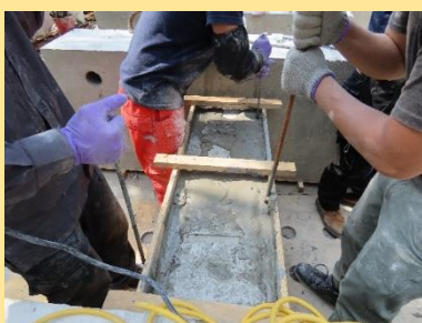
(e)補強層澆置UHPC
