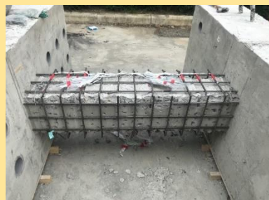
(c)固定鋼筋網
