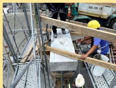
(e)補強層澆置UHPC
